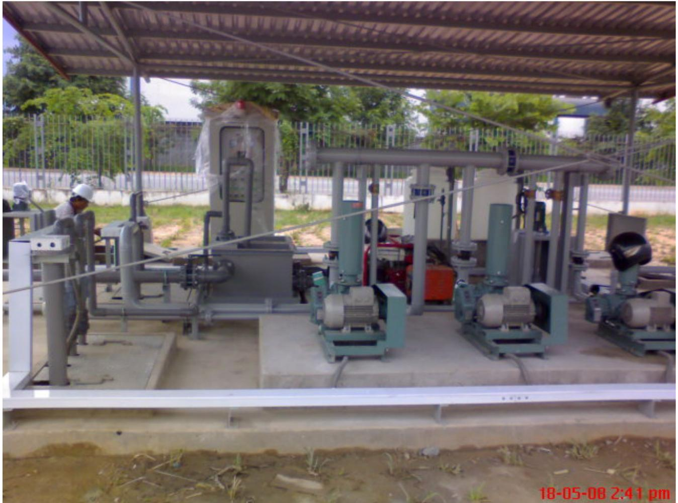
Sewage Waste Water Treatment Plant Capacity 5m<sup>3</sup>/h
